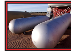
2 1000 Gallon LP Tanks converted to diesel
